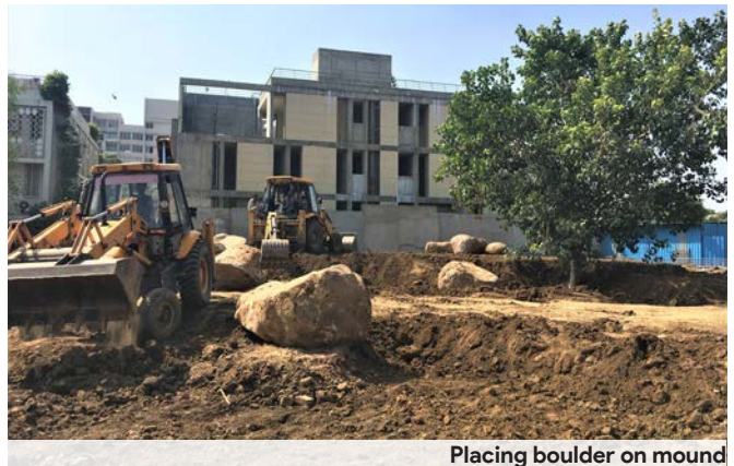
Placing boulder on mound
